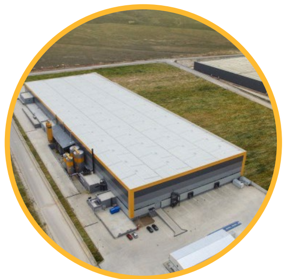
ODE Eskişehir, Turkey Production Facilities
