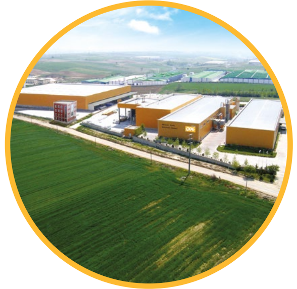
ODE Çorlu/Tekirdağ, Turkey Production Facilities
