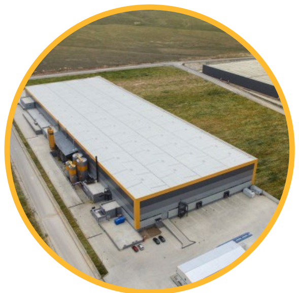
ODE Eskişehir, Turkey Production Facilities
