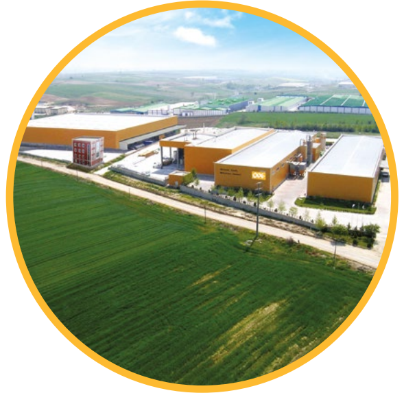
ODE Çorlu/Tekirdağ, Turkey Production Facilities
